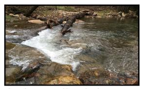
A newly constructed log and rock cross vane. in the South Fork of Bens Creek mitigation
